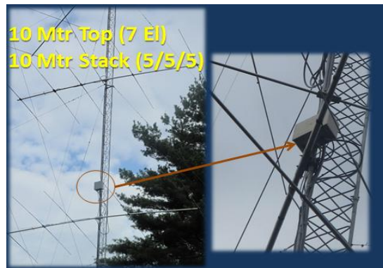
Stacked Yagis on 10 - Meters
